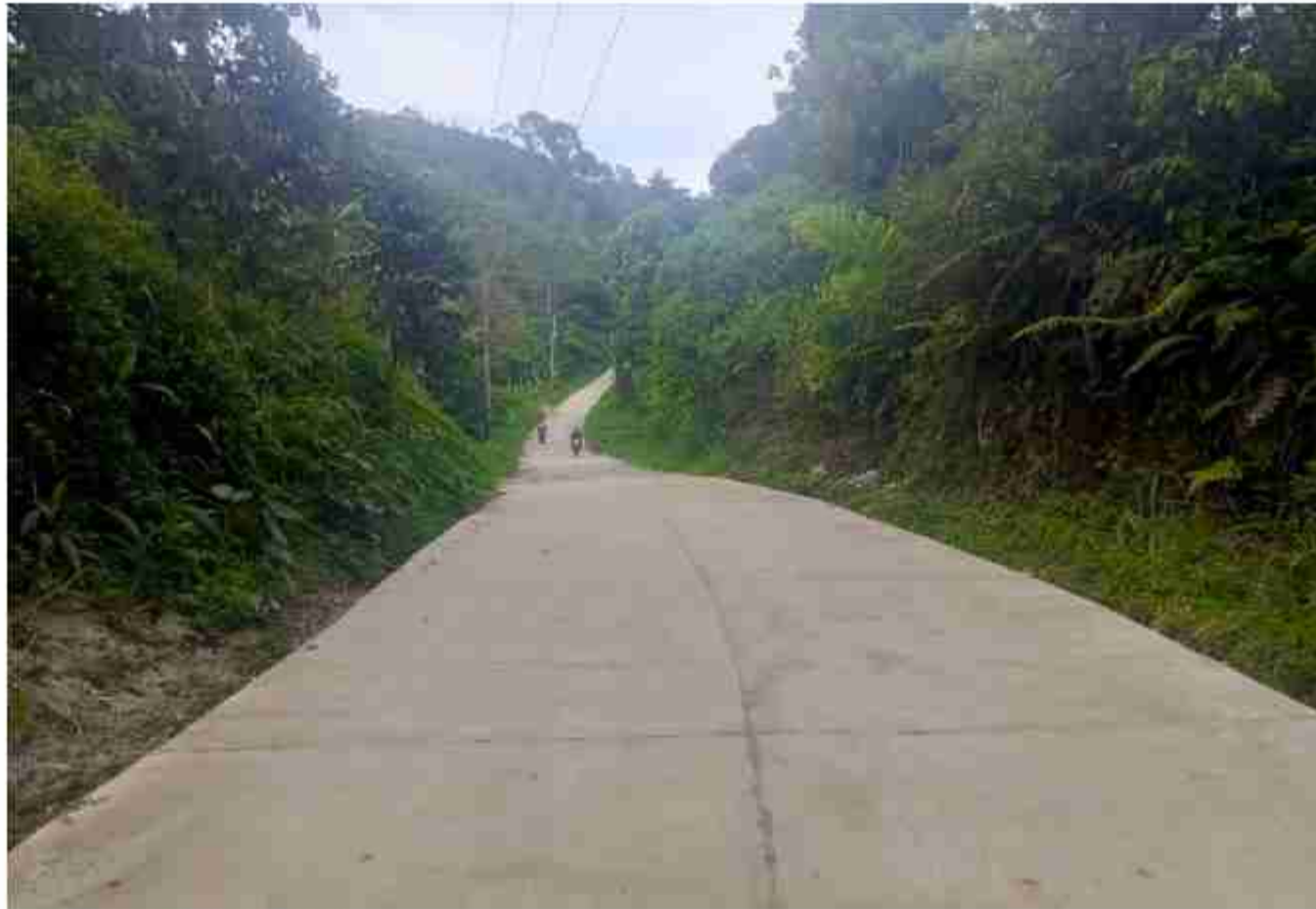
Gambar 4.3 Ruas Jalan Suoh
